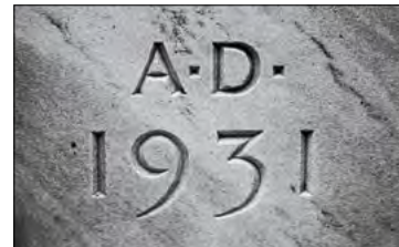
The building's cornerstone.
